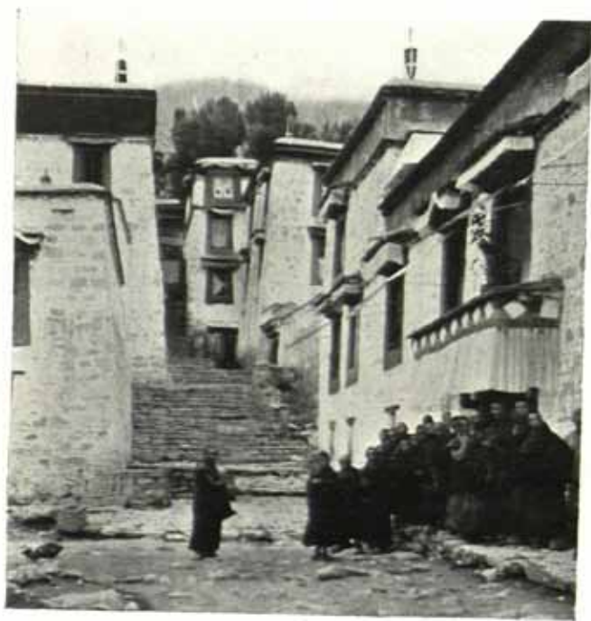
CORNER OF COURTYARD OF ASTROLOGER'S TEMPLE, NECHANG.
