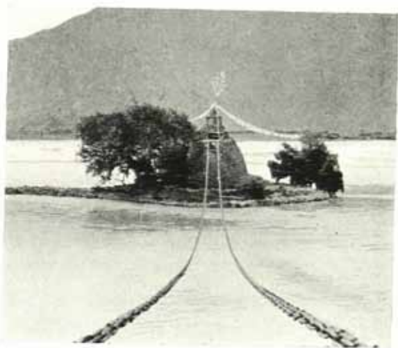
OLD CHAIN BRIDGE AT CHAKSAM.
